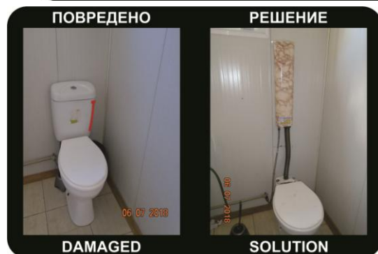
Cracked mono-block replaced by a cistern in the Blue Zone - Yambol
